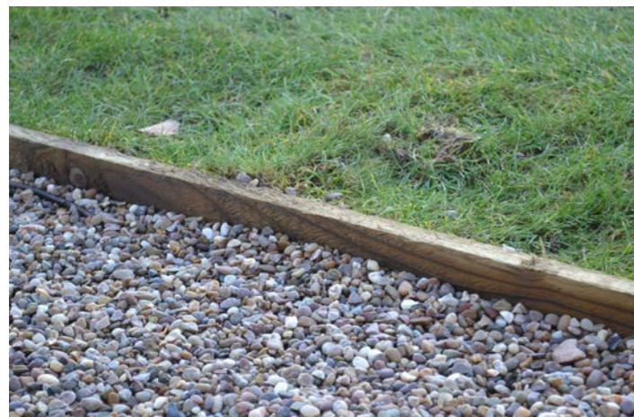
Loose gravel & timber edge - Allotments
