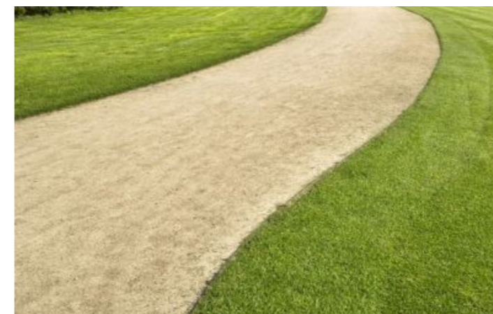
Self-binding gravel pathways - Secondary circulation (3m)
