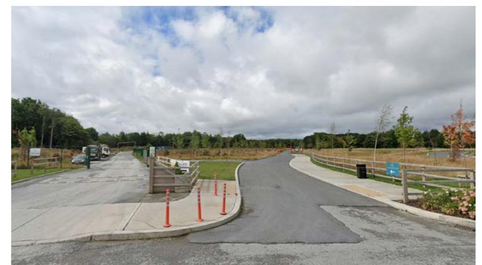
Figure 20: Main entrance into the site.
